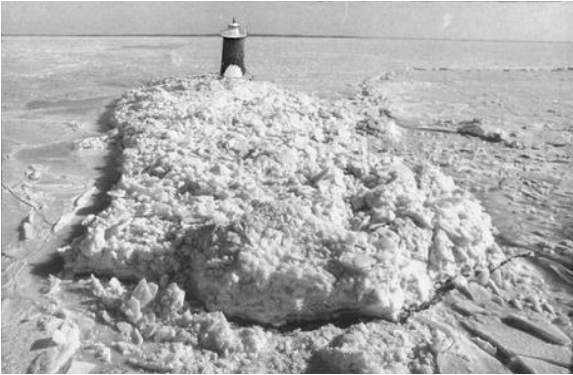
Figure 15. The power of the flowing Chesapeake ice can be seen in this 1977 photo showing ice piling up around the Sharps Island lighthouse. Prior to the winter of 1977, the lighthouse was vertical. After the winter of 1977, the lighthouse's caisson structure, which sits in ten feet of water, was sharply tilted.
